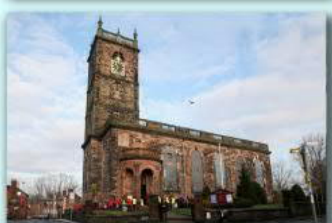
St Alkmund's Church The medieval church collapsed in 1711. A new church was quickly erected. Built of brick and faced with stone, it was consecrated in 1713.
